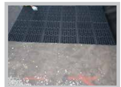
Fig. 18 Maintain 12" overlap on textile.
