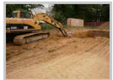
Fig. 4 Excavate according to plans, following all governmental regulations.
