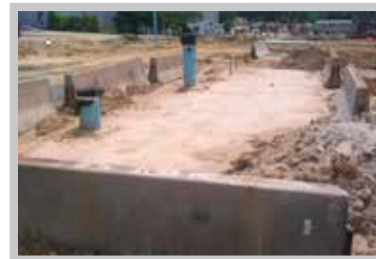
Fig. 28 Secured R-Tank® installation using Jersey Barriers.
