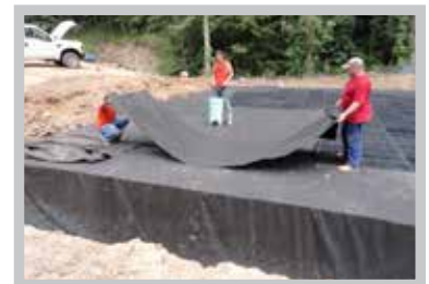
Fig. 20 Encapsulate R-Tanks® with geotextile.
