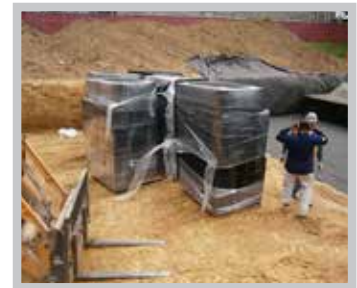
Figure 3 Installation can be sped up by either assembling the tanks in the excavation or placing the pre-assembled tanks in the excavation.
