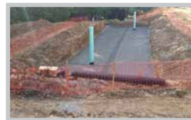
Fig. 27 Secure the installation with temporary fencing.
