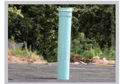
Fig. 16 Installed maintenance port
