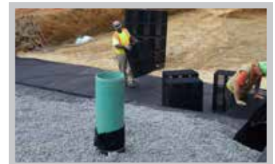
Fig. 11 Installed Inspection Port
