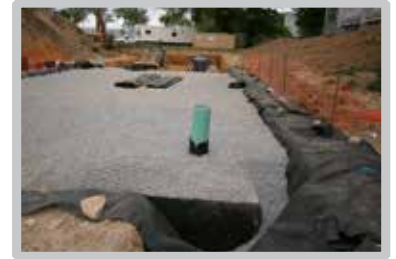
Fig. 24 Use an LGP dozer to push backfill over R-Tank® units.
