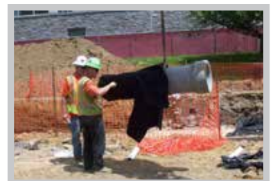
Fig. 22 Seal the pipe boot with the included band clamps and duct tape.
