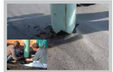
Fig. 19 Cut an "X" into textile to accommodate pipe penetration and seal with a boot.
