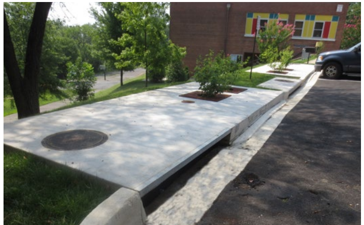
StormGarden with a pre-treatment chamber
