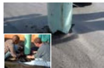
Fig. 19 Cut an "X" into textile to accommodate pipe penetration.
