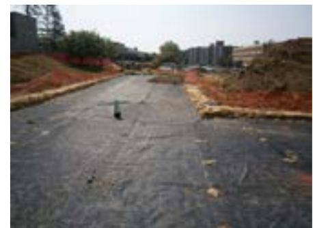
Fig. 25 Overlap Geogrid 18" or as required by plans.
