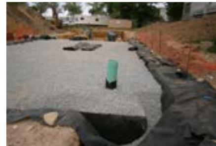
Fig. 24 Use an LGP dozer to push backfill over R-Tank<sup>HD</sup> units.
