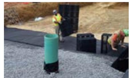
Fig. 11 Installed Inspection Port
