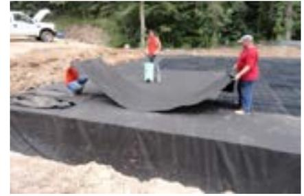
Fig. 20 Encapsulate R-Tanks<sup>HD</sup> with geotextile.
