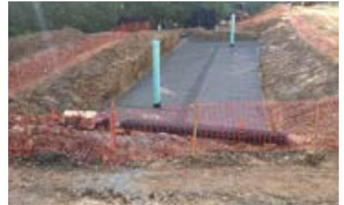
Fig. 27 Secure the installation with temporary fencing.
