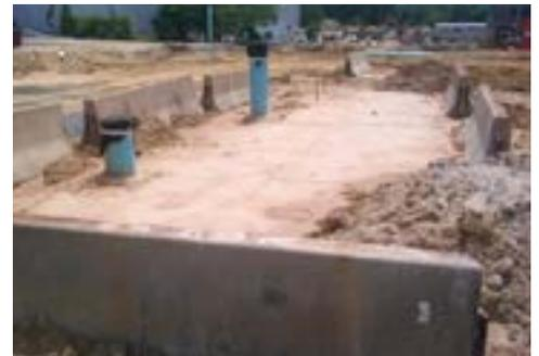
Fig. 28 Secured R-Tank<sup>HD</sup> installation using Jersey Barriers.
